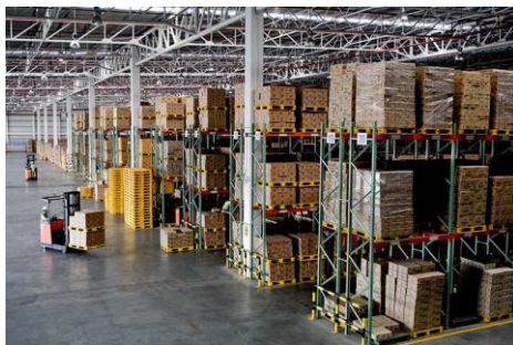
Fig 2. Storage Facility in Detroit
